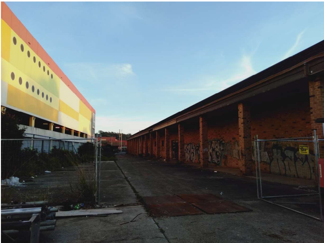
Photograph 4: The concrete driveway between the two buildings.
