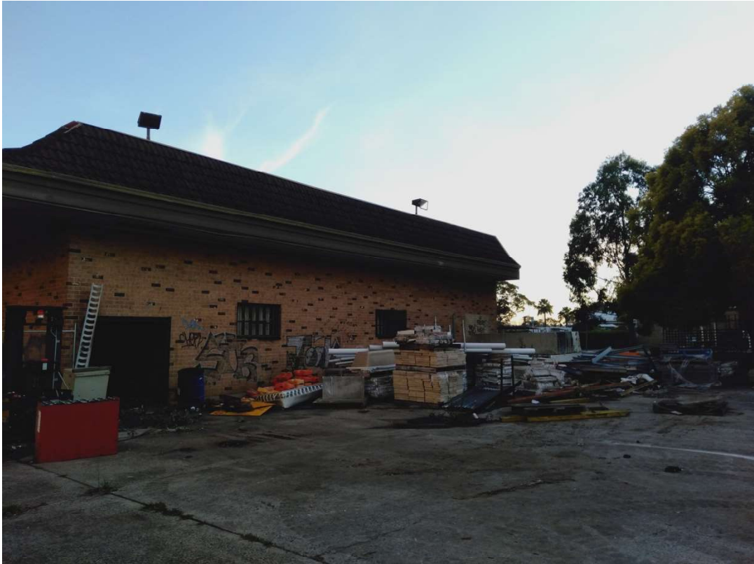
Photograph 3: The rear of the brick storage building (the south-eastern portion of the site).
