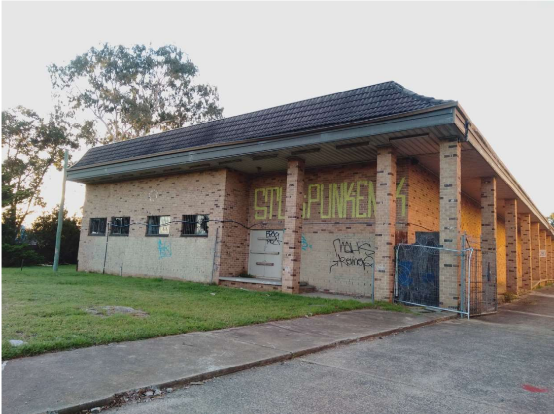
Photograph 1: The brick storage building (former tenpin bowling centre) at 24 Queen Street.
